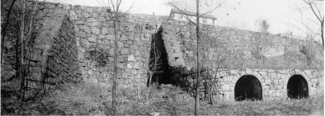
**Figure 18.** Undated (partial) view of the stone foundation with arches believed to be part of the trestle system that carried rail cars to the filling house and first nail factory. Note the stone wall behind that held up the Morris Canal above.<sup>18</sup>
