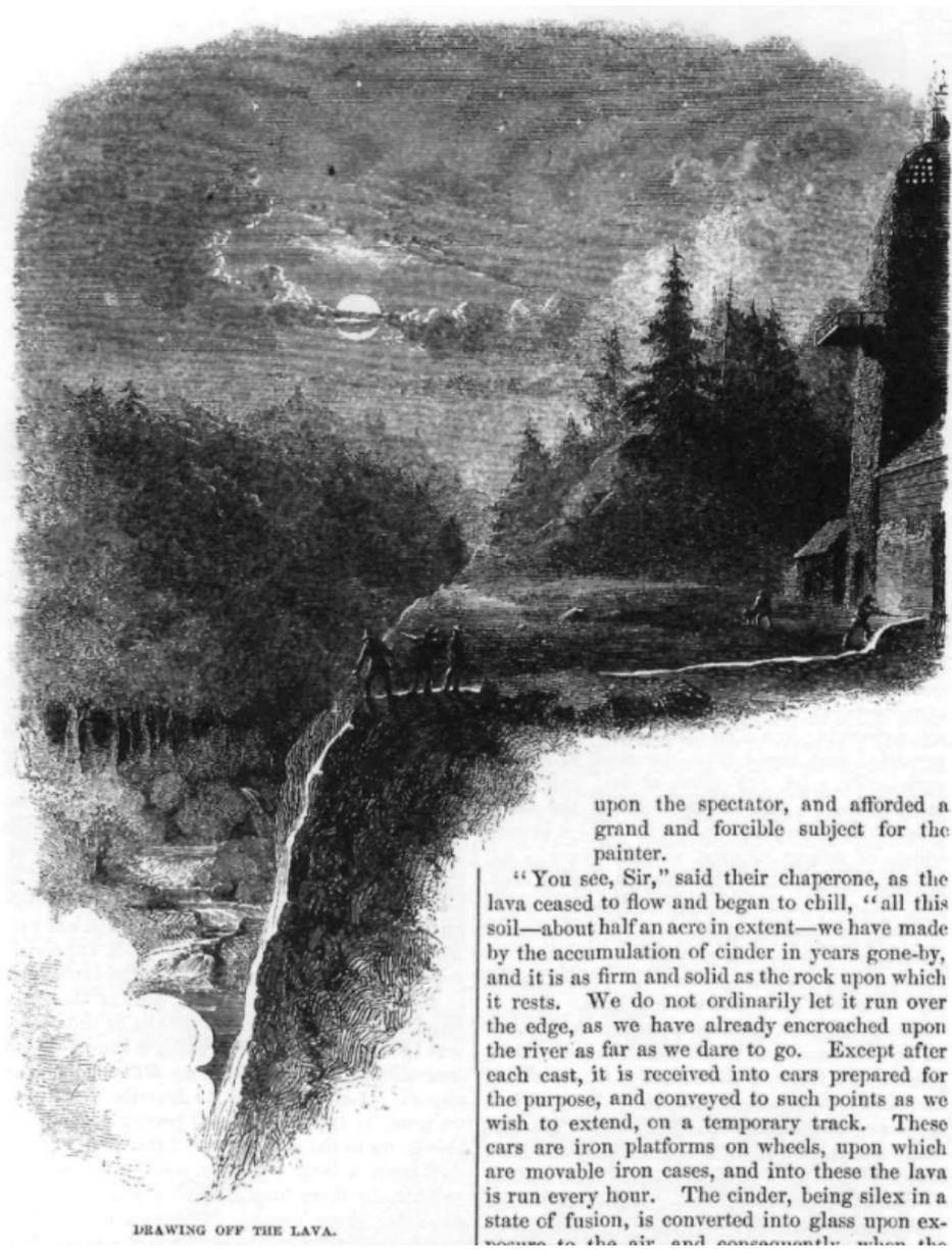
Figure 31. Drawing depicting the drawing off of the slag from the blast furnace into the Rockaway River in the 1860 article “Among the Nail-Makers” in *Harper’s New Monthly Magazine*.<sup>31</sup>
