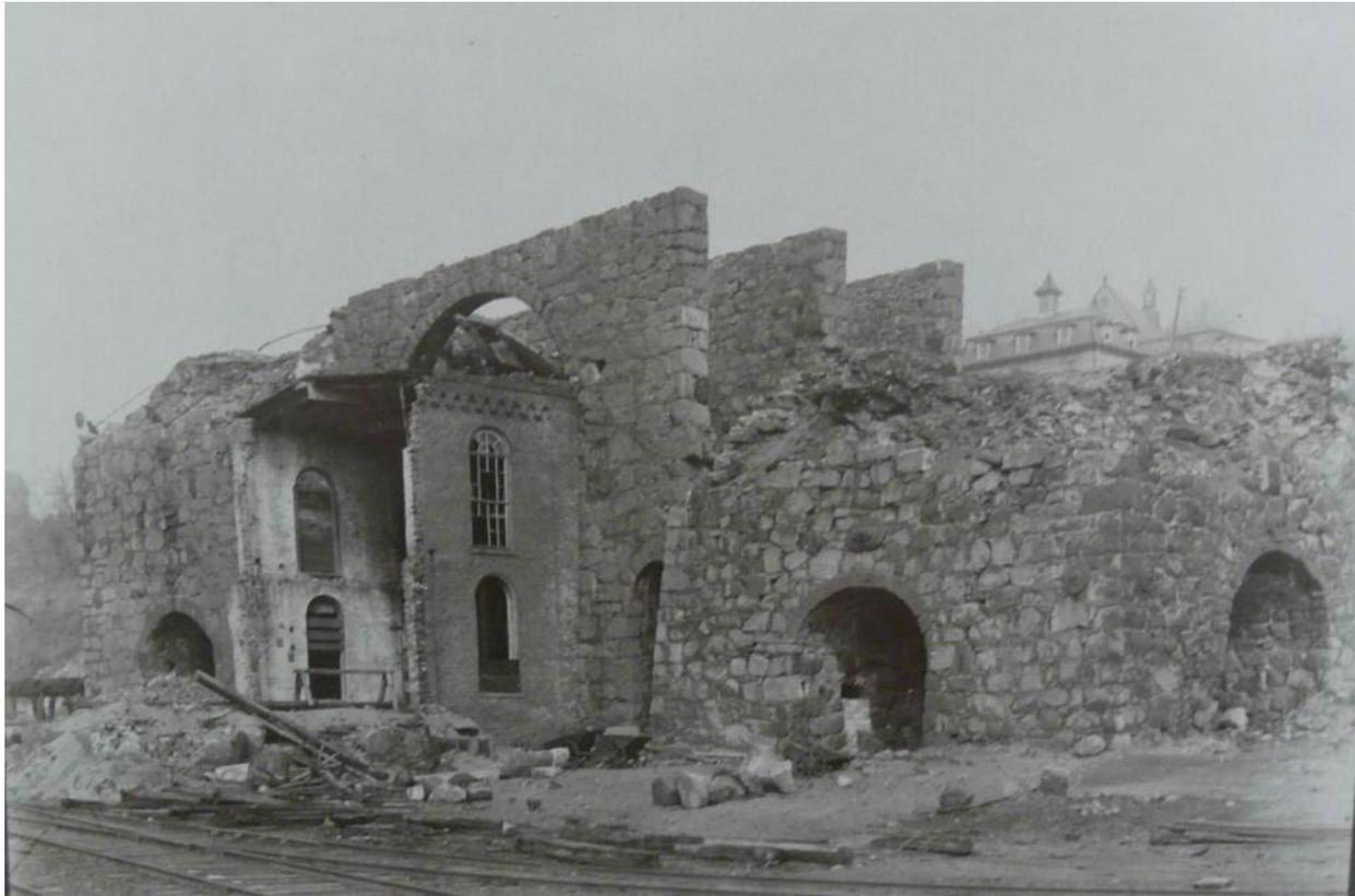
**Figure 22.** Circa 1890s image of the blast furnaces being dismantled.<sup>22</sup>
