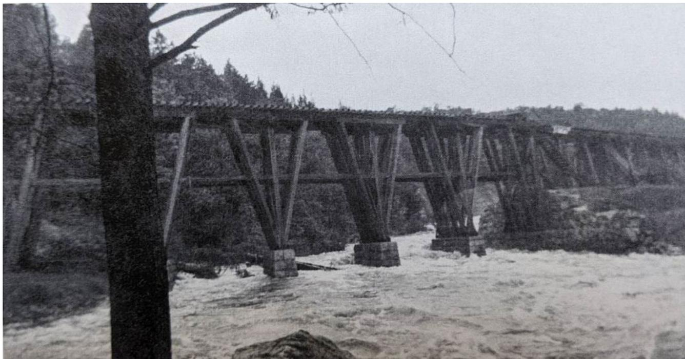
**Figure 16.** Undated (pre-1896) view of the original wooden railroad trestle when the river was high at flood stage. Note the rubblestone retaining walls along the river banks that were incorporated into the 1906 steel railroad trestle that replaced the wooden one.<sup>16</sup>
