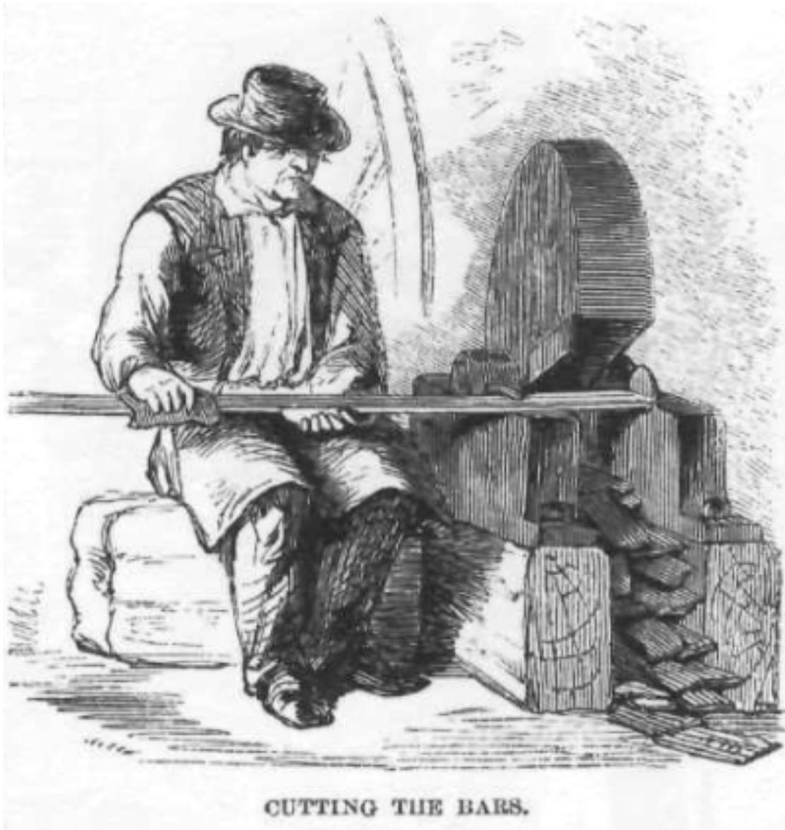
**Figure 37.** Drawing depicting a worker cutting bars in the 1860 article “Among the Nail-Makers” in *Harper’s New Monthly Magazine*.<sup>37</sup>
